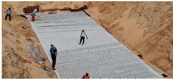
Boys Block STP works
